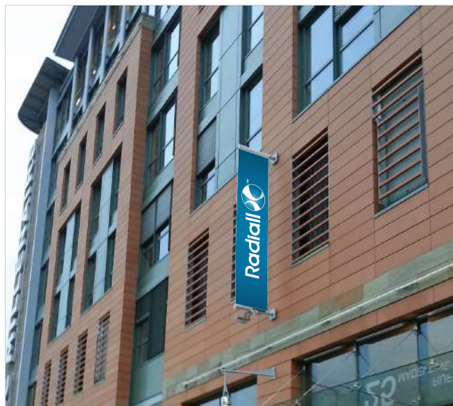
Head office - Aubervilliers France
